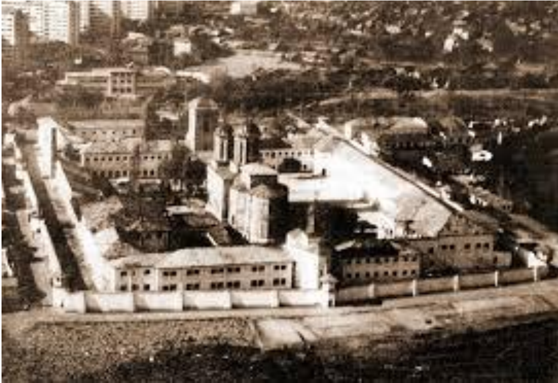
FIG 14 The avoidable demoltion of Vacaresti Monastery
