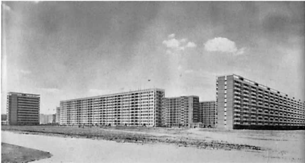
Balta Albă housing district, Bucharest, Romania. Photograph (uncredited). Illustrated in Arhitectura 101, no. 4 (1966): 32.
