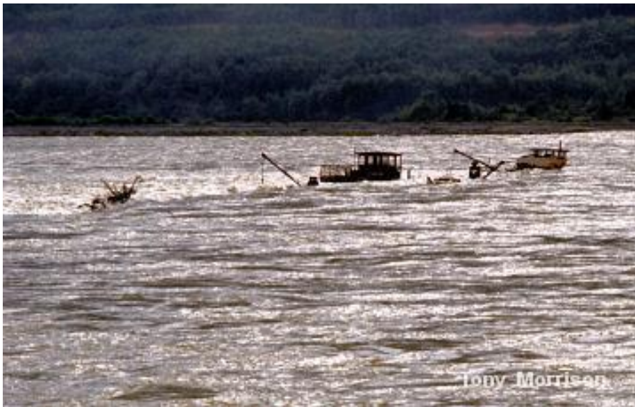
Fig 6 The Iron Gates – wrecks and new road construction in 1966
